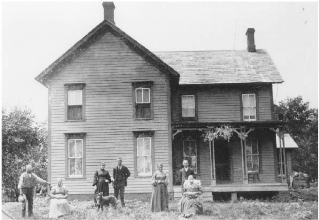
The Jackson Hull Family With View of the House Built in 1878
